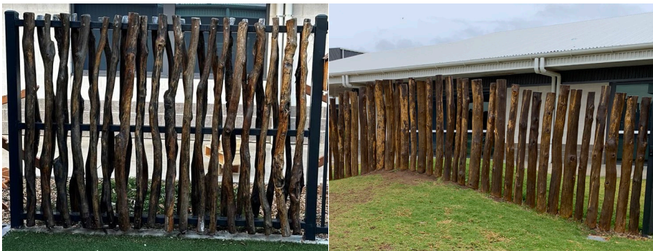
Figure 8: Example of feature fencing requiring entrapment risk compliance.
